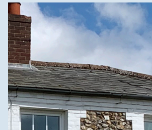
Slate tile roof
