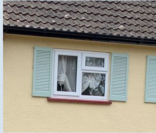
Window with external shutters
