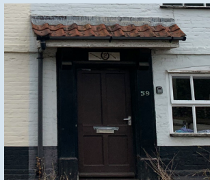
Flat roof porch feature
