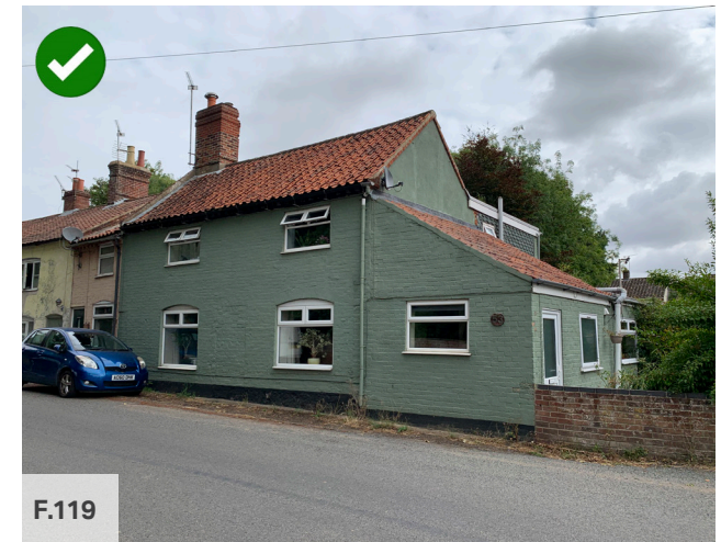
Figure 119: Side extension which complements the scale of the existing property
