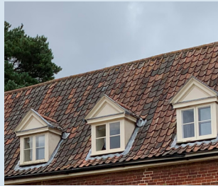
Gabled roof dormer
