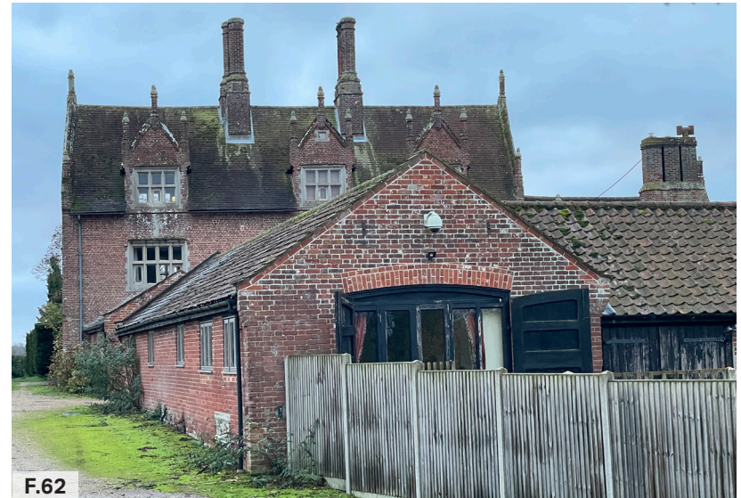
Figure 62: Rear elevation of Hautbois Hall
