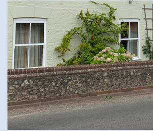
Gault brick wall
